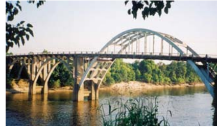
Edmund Pettus Bridge over the Alabama River at Selma
