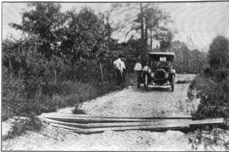
A DANGEROUS CULVERT.
