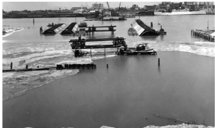
Construction of Bankhead Tunnel
