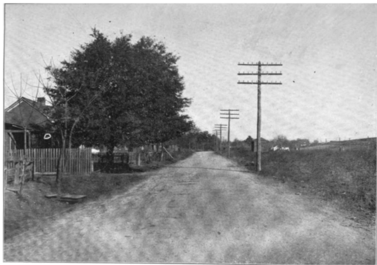
Gravel road, Montgomery County, near City of Montgomery. This road is ten years old. It has been scarified, several inches of Lafayette gravel added and resurfaced with road machine.
