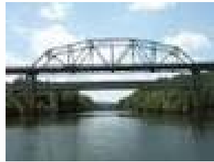
Mulberry Fork Bridge over the Warrior River near Jasper, Alabama
